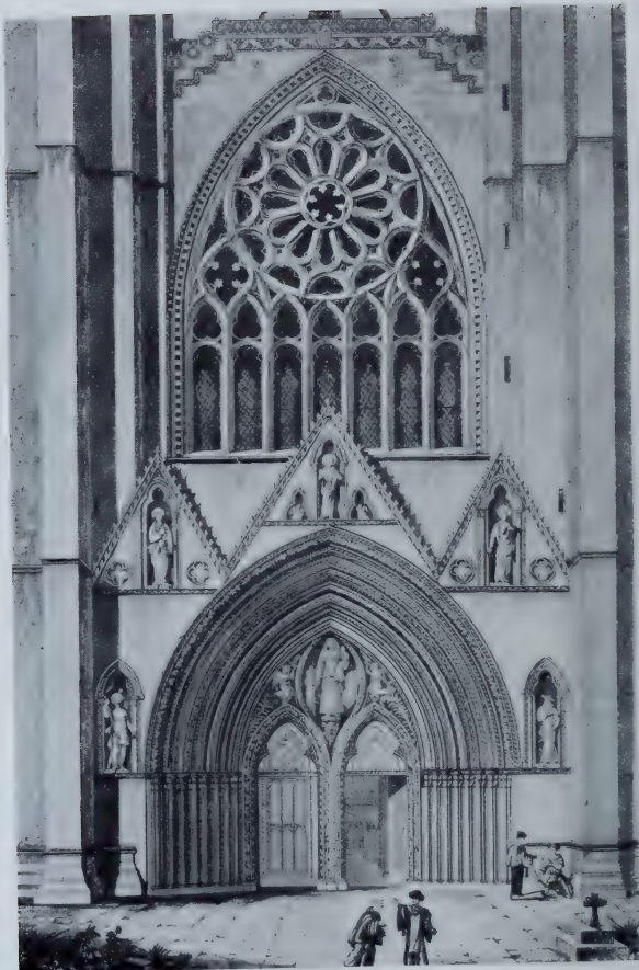
The Cathedral. Grand Entrance restored.
