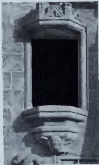
FIG. 4.—A “made-up” Photograph showing how the Stones of this charming little Oriel Window should have been arranged.
